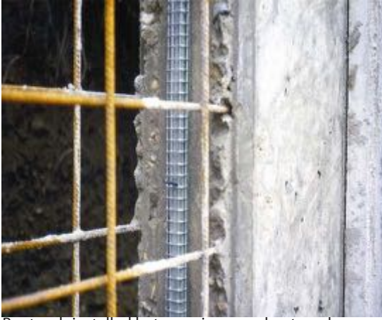
Bentorub installed between inner and outer rebar, with Bentosteel wire mesh
